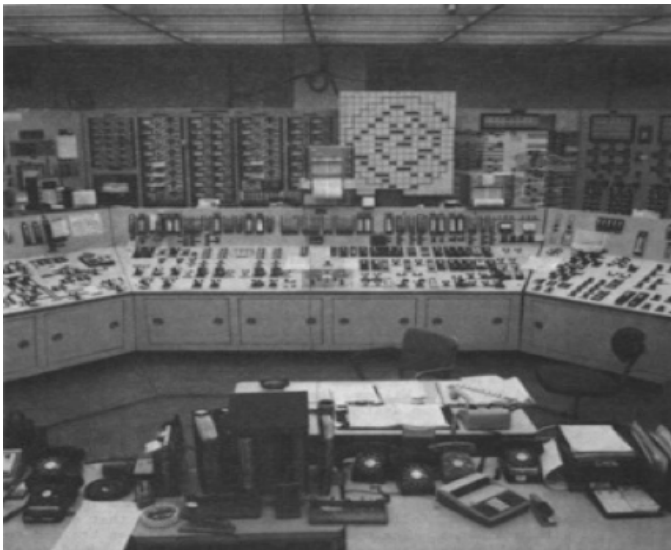
Figure 1. Three Miles Island control room (Kenemy, 1979, p.112).
